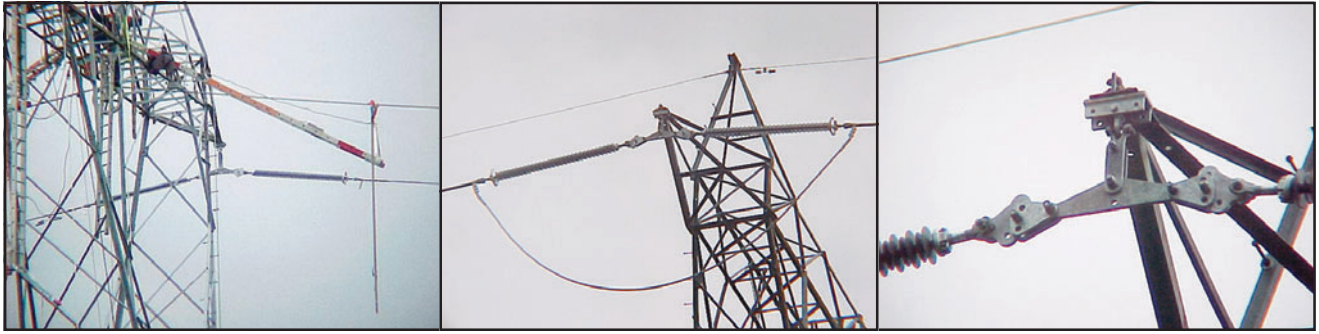
The “special” yoke plate, connecting the two strain assemblies.
