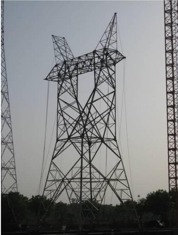
Deadend Structure passed all loading without a failure
