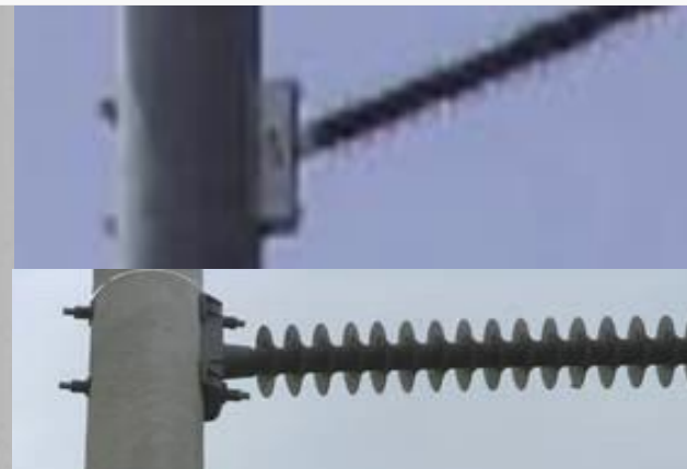
FLAT BASE (2 BOLT CONNECTION) 1.1-2.5 \cdot 10^5 Nm/rad
