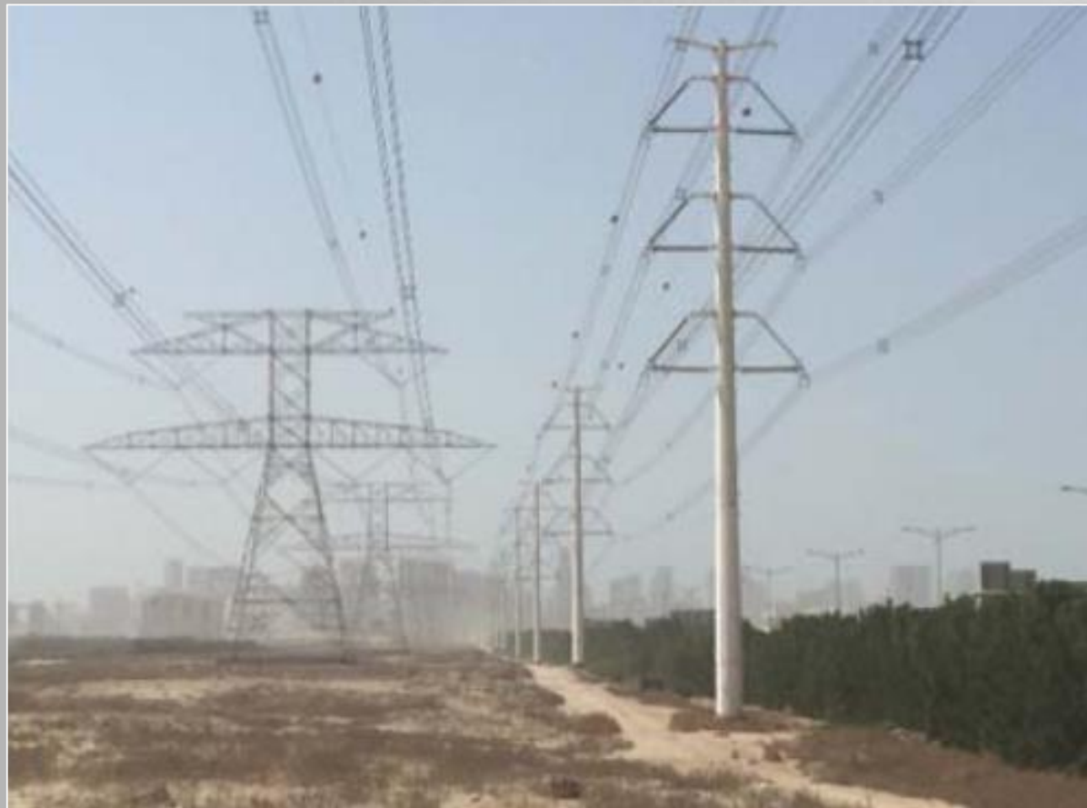
Traditional vs Compact Double circuit 420 kV lines in Dubai.
