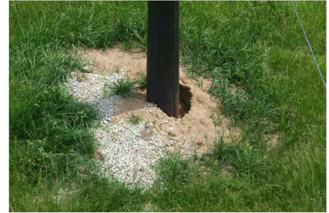
Figure 6-2. Direct embedded pole.
