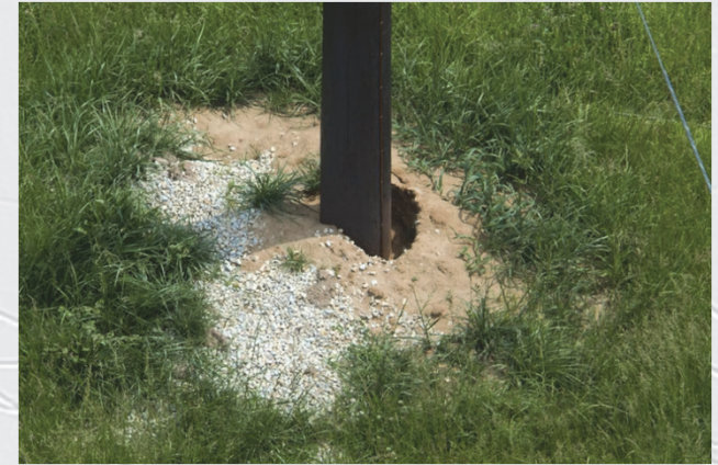
Figure 6-2. Direct embedded pole.
