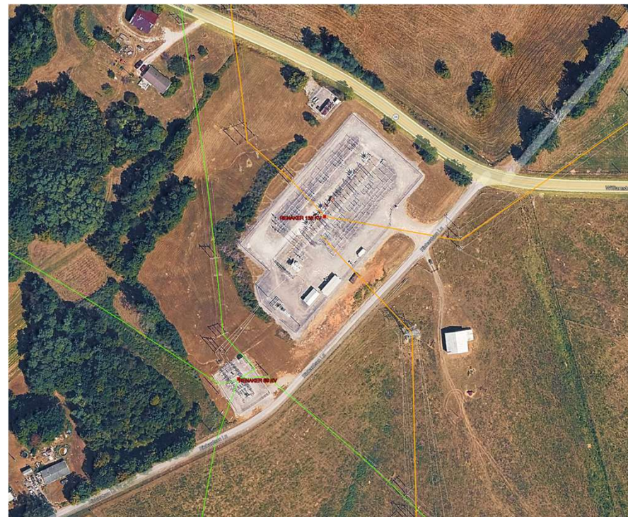
Renaker Substation - After
