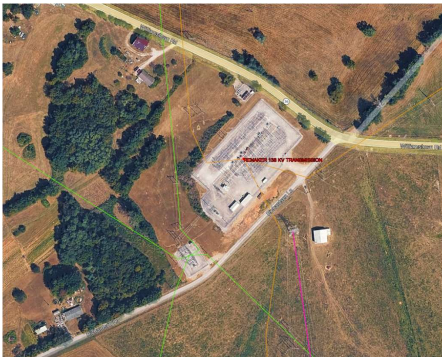
Renaker Substation - Before
